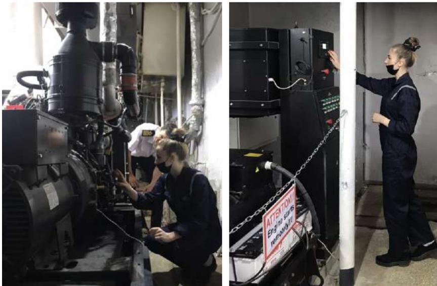
**Figure 3.** Participant in the real conditions preparing to start and start of emergency diesel generator in the academic engine room laboratory
